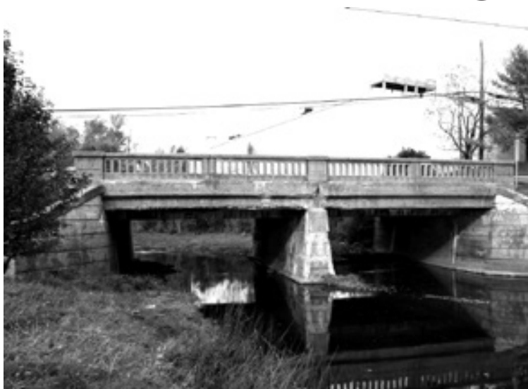
The present bridge over Flat Run was built in early 1912, replacing a much older wooden bridge.
