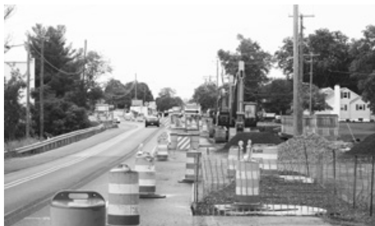
The year long nightmare on Main Street is about to begin.
