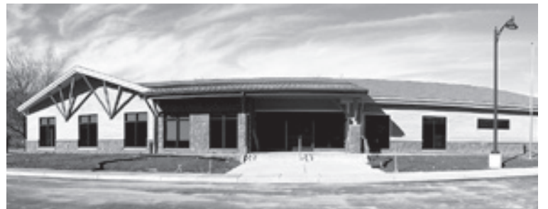
The new Carroll Valley Borough building opened its doors for business on March 1. This new building houses the Borough offices, the Fairfield branch of the Adams County Library and the Carroll Valley Police Department.
