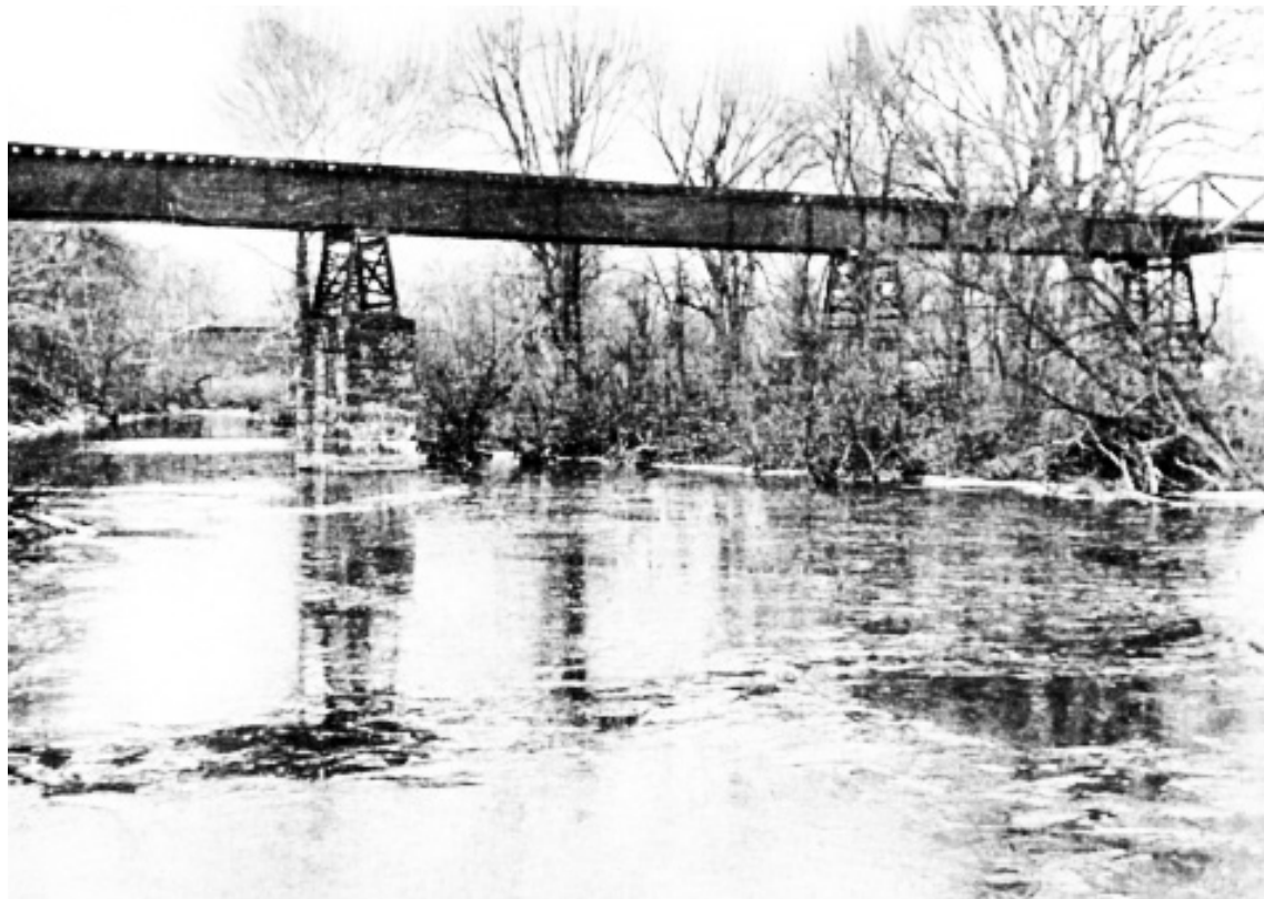
Emmitsburg Railroad bridge over Toms Creek. The center pylon is still visible today, just south of the current bridge over the creek.
